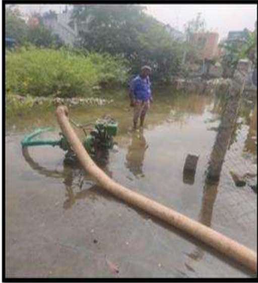
BAILING OUT WATER USING DIESEL ENGINE AT ST.THOMAS STREET, ZONE -1 (WARD NO:18)
