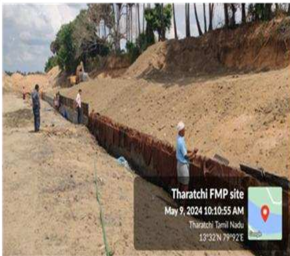
Proposed Flood protection wall @LS 69.00Km during execution
