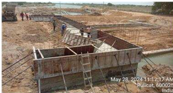
Left Abutment, Wing and return wall
