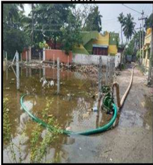
BAILING OUT WATER USING DIESEL ENGINE AT SCHOOL STREET, ZONE - 1 (WARD NO:19)
