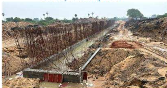
RCC Wall 1st Lift
