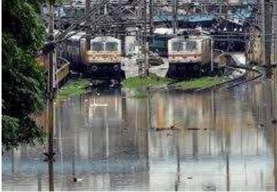
Flood inundation in Railway track at Avadi
