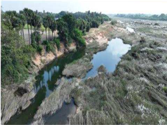
Breach portion in Left Side Flood Bank at LS 69.00Km during flood
