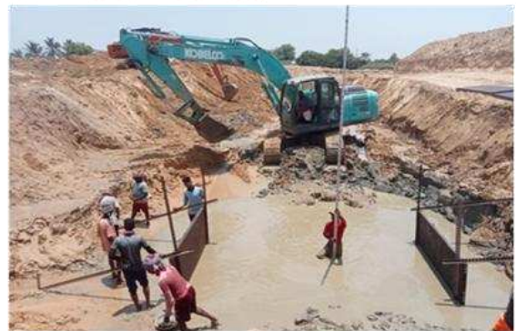
Earthwork excavation for Foundation
