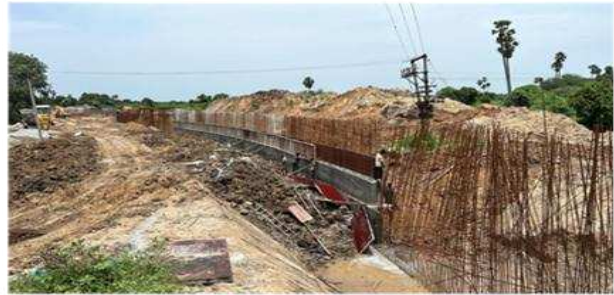
RCC Retaining Wall 5 th lift
