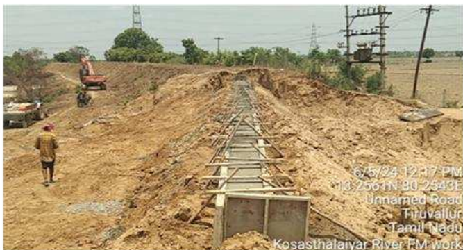
Corewall construction - Concreting
