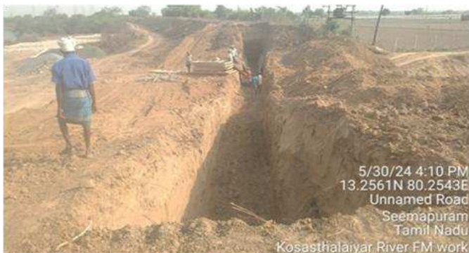
Corewall construction - Earthwork
