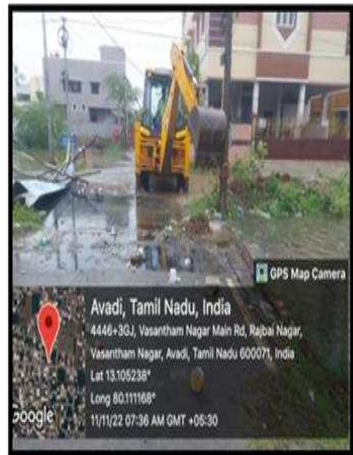
DESILTING USING JCB NEHRU NAGAR CHURCH STREET, ZONE -1 (WARD NO:18)
