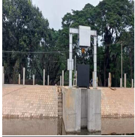
Right Side of Sluice Work
