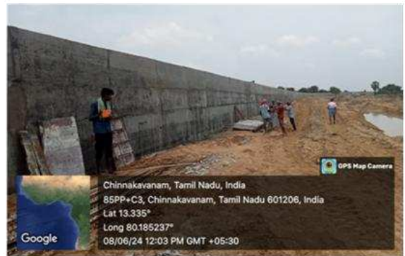
RCC Retaining wall
