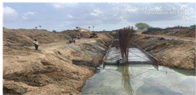
RCC Retaining Wall base slab
