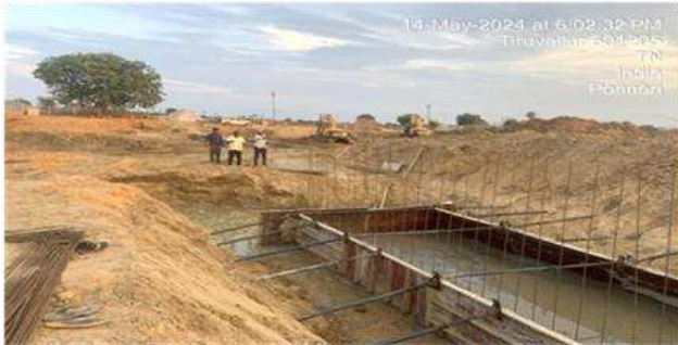
Left side Guide wall 1st lift
