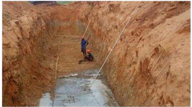
PCC Levelling course
