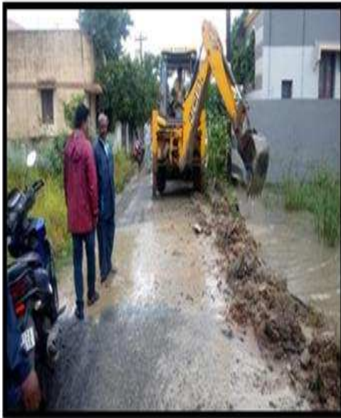
DESILTING USING JCB AT VASANTHAM NAGAR, ZONE -3 (WARD NO:43)
