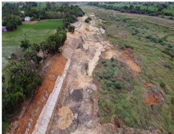
Flood protection wall @LS 69.00Km during execution
