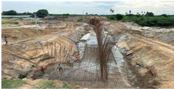
RCC Retaining wall reinforcement
