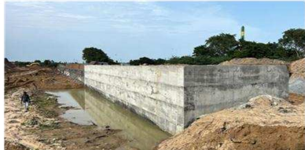
RCC Retaining Wall
