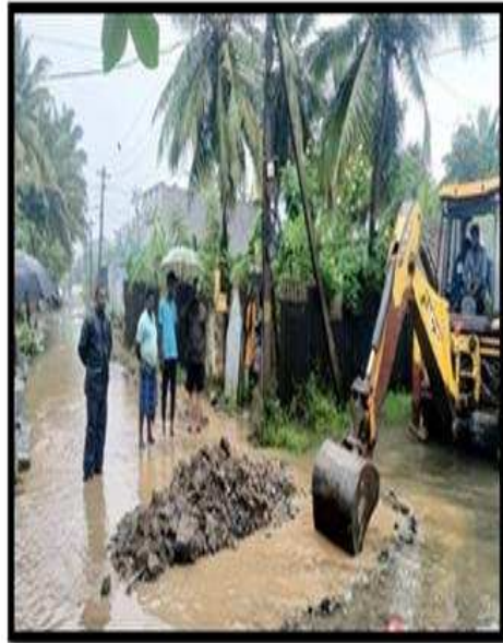
DESILTING USING JCB AT THULASI STREET, ZONE -4 (WARD NO:38)
