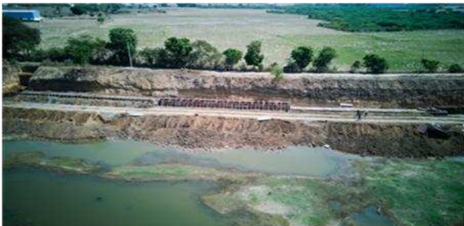
Flood protection Wall construction in Left Side Flood Bank
