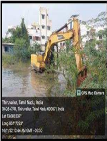
DESILTING USING JCB AT REVA NAGAR, ZONE - 3 (WARD NO:48)
