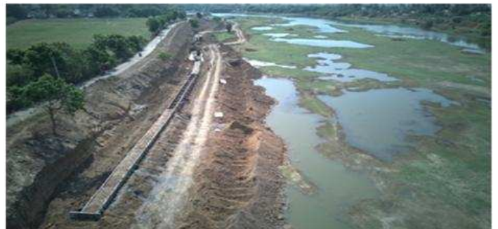
Flood protection Wall construction in Left Side Flood Bank
