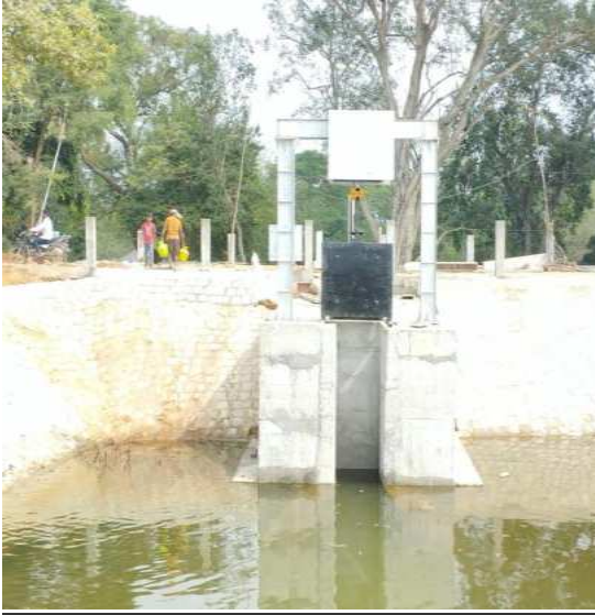
Left Side of Sluice Work
