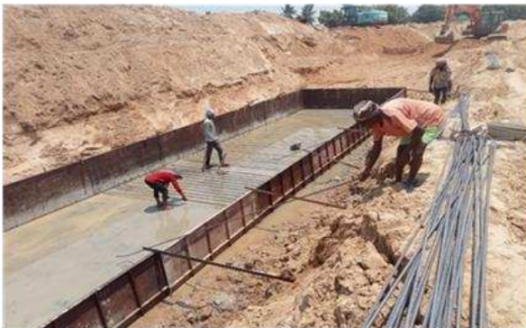
Steel Reinforcement tying for retaining wall
