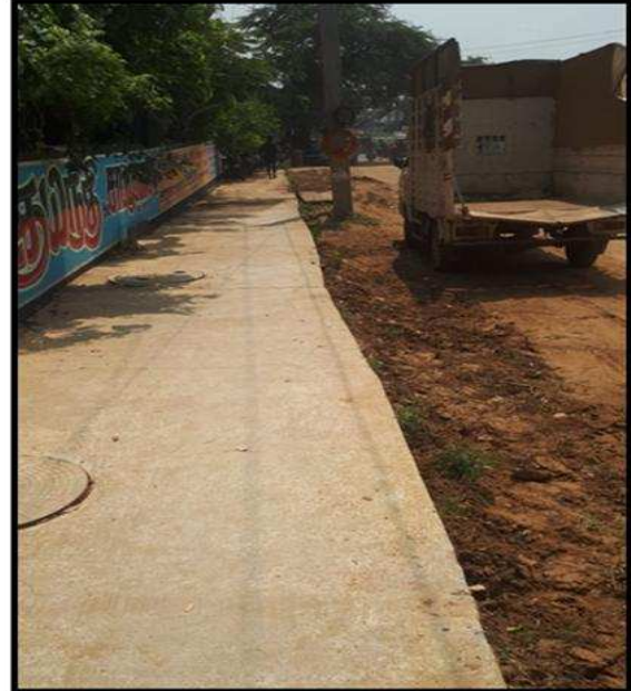
Construction of SWD and Culvert at IAF Main Road in Ward no 15
