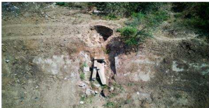
Damaged Inlet
