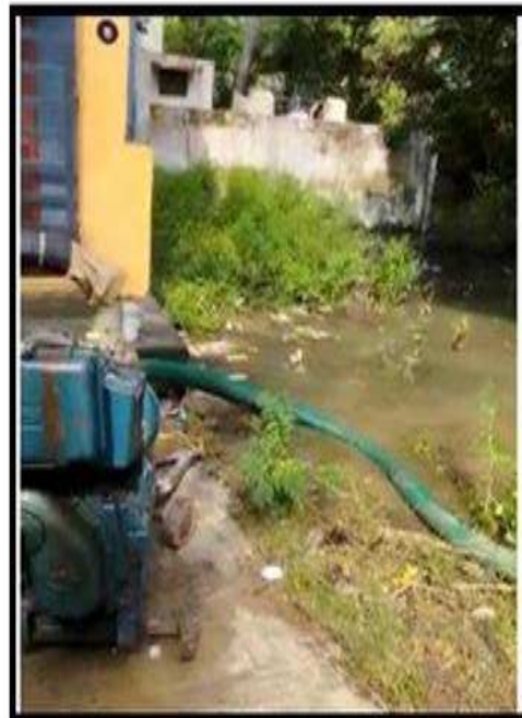
BAILING OUT WATER USING DIESEL ENGINE THULASI STREET, ZONE -4 (WARD NO:38)
