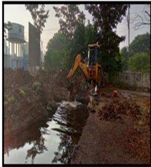
DESILTING USING JCB AT THULASI STREET, ZONE -4 (WARD NO:38)
