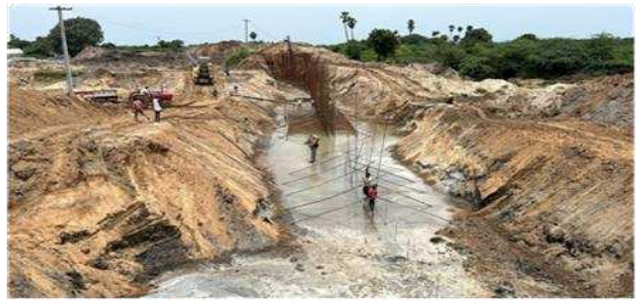
RCC Retaining Wall base slab
