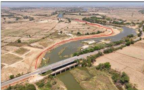
RCC Retaining Wall alignment
