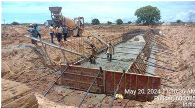
2 nd lift Concrete
