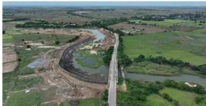
THATTAMANJI Flood Protection wall Work During Execution
